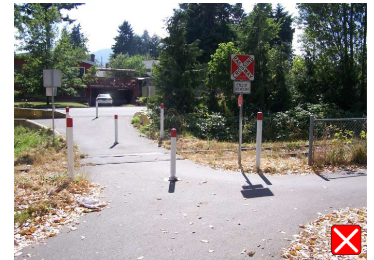
This crossing was disliked because there was no cross marking and appeared unsafe for trail users
